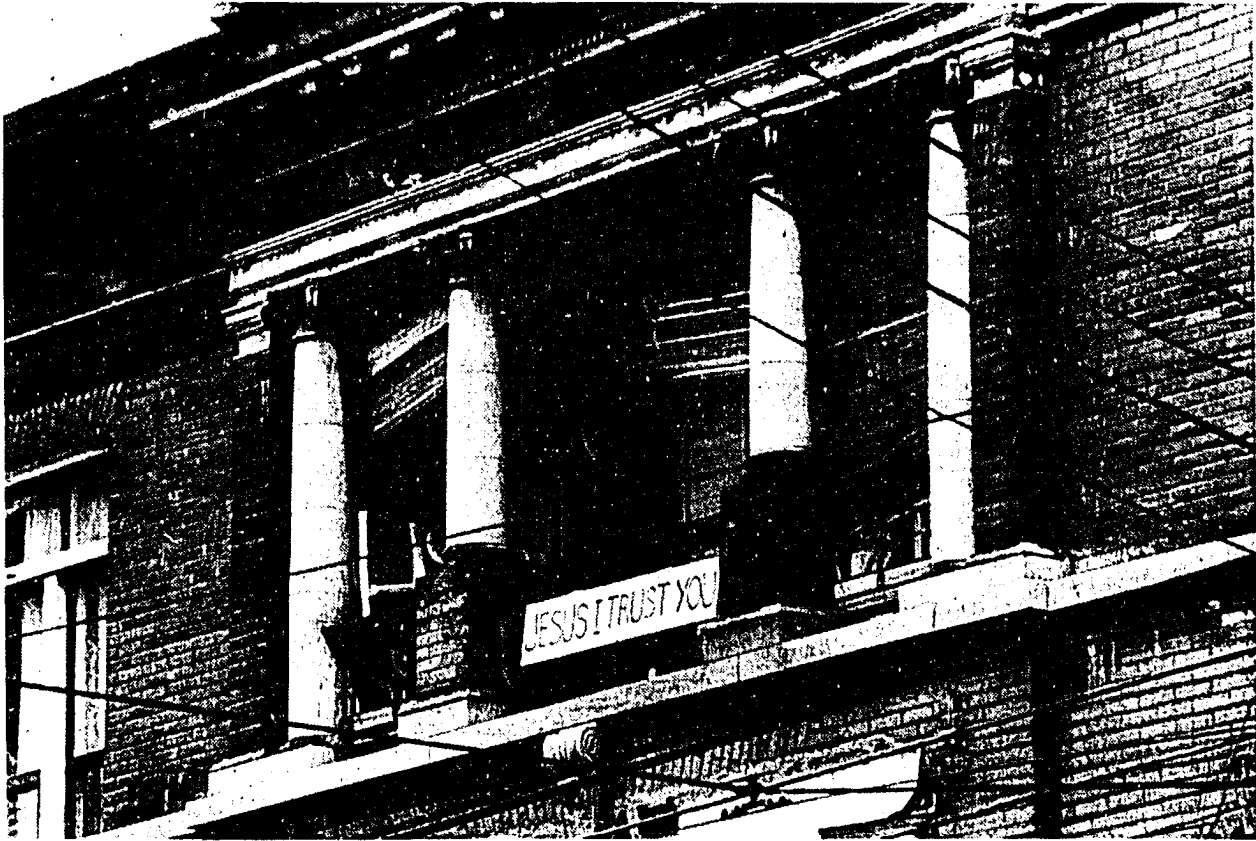
Toronto's Parkdale district: some of the structures on this strip of Queen West date from as early as the 1860s.
