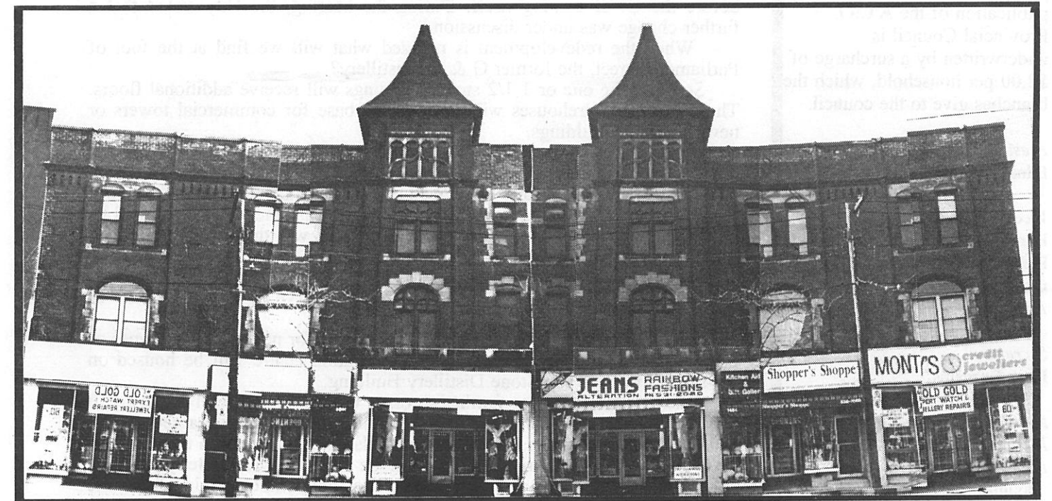
A view of the historic streetscape on the south side of Queen Street West at Macdonnell and Lansdowne Avenues.
