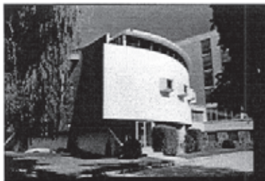
The Ontario Bible College on Ballyconnor Court designed by Peter Dickinson.
