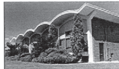
St Louie di France designed by Mendelow, Keywan and Henry Fleiss on Don Mills Road.
