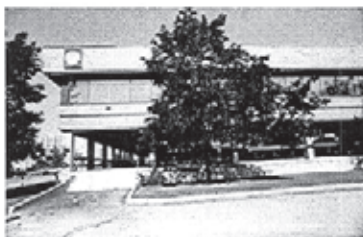
The Shell Canada Building on 75 Wynford Drive designed by Webb, Zerafa and Menkes.
