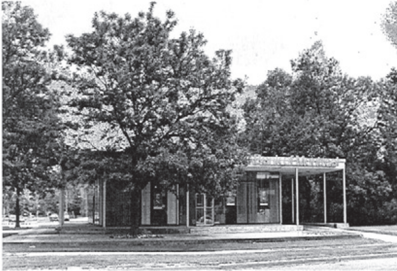
The Bank of Montreal is a pure example of the clean lines and precision of Modernism.
