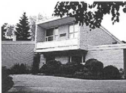
The upper level of the Betel residence angles up and projects over the front entrance.
