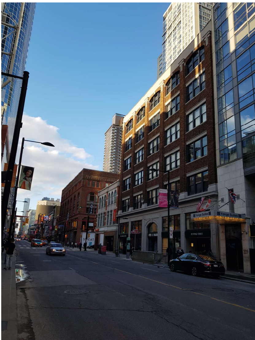
The Adams building and its adjacent buildings (Own source, 2019).
