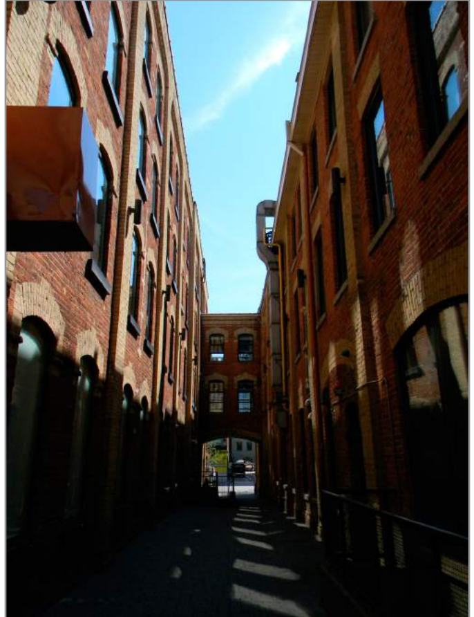
Laneway in King-Spadina, used as a mid-block connection
