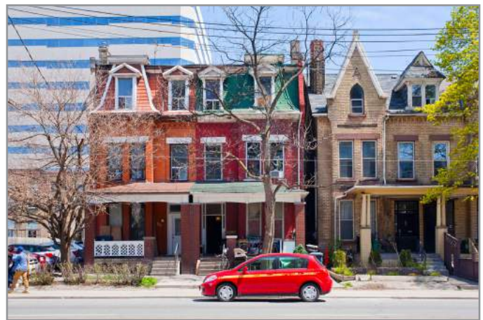
Representative example of the residential building typology
