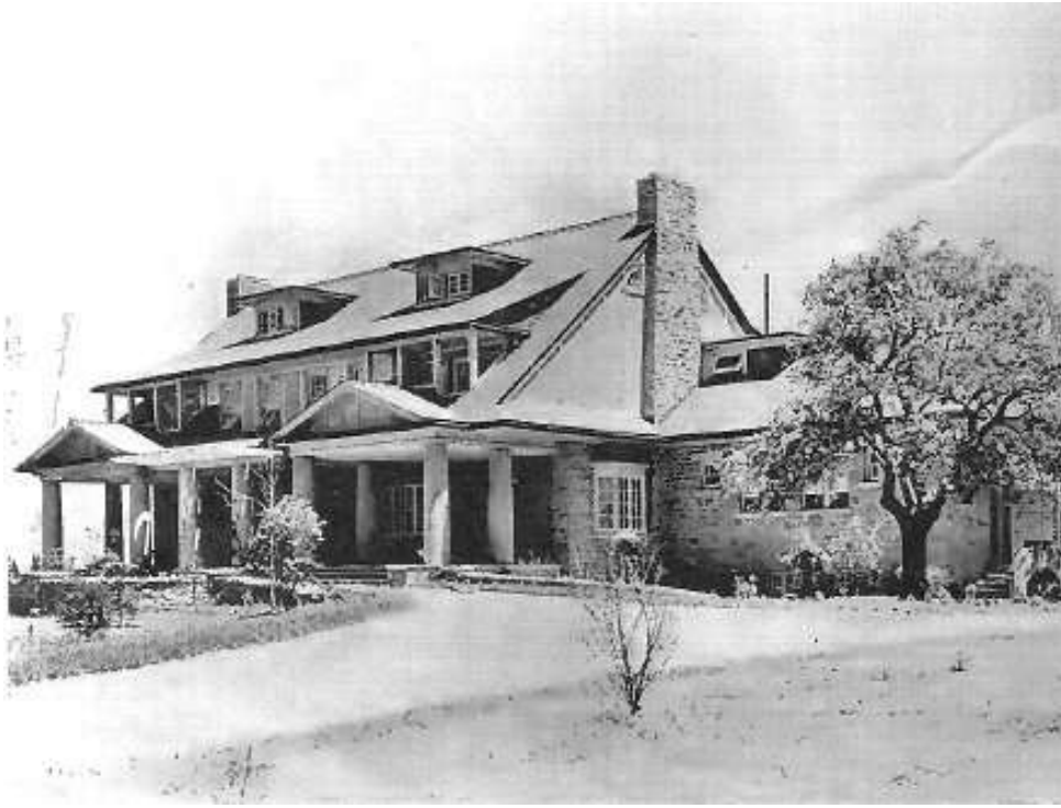
12 East façade of Ormscliffe as designed by F.H. Herbert, published in “Residential Design in Canada,” Construction , vol. 4, no. vii (July 1910), pp. 112-113.
