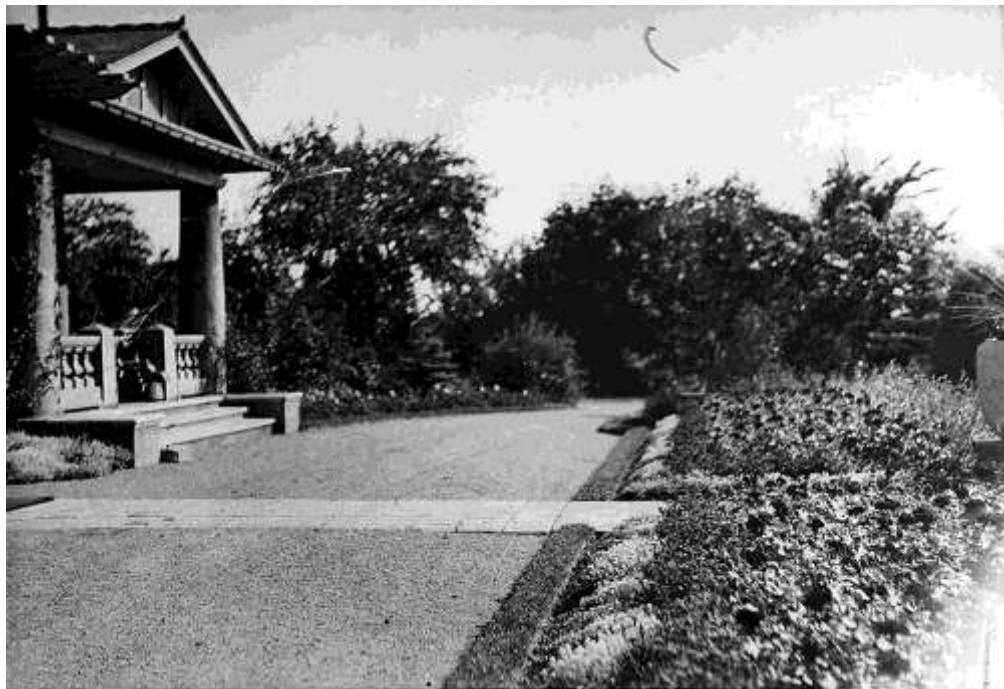
13 Detail of the driveway terrace at Ormscliffe in 1911, with the original arrangement of the open verandah. ( City of Toronto Archives, Fonds 1244, Item 3109 ).
