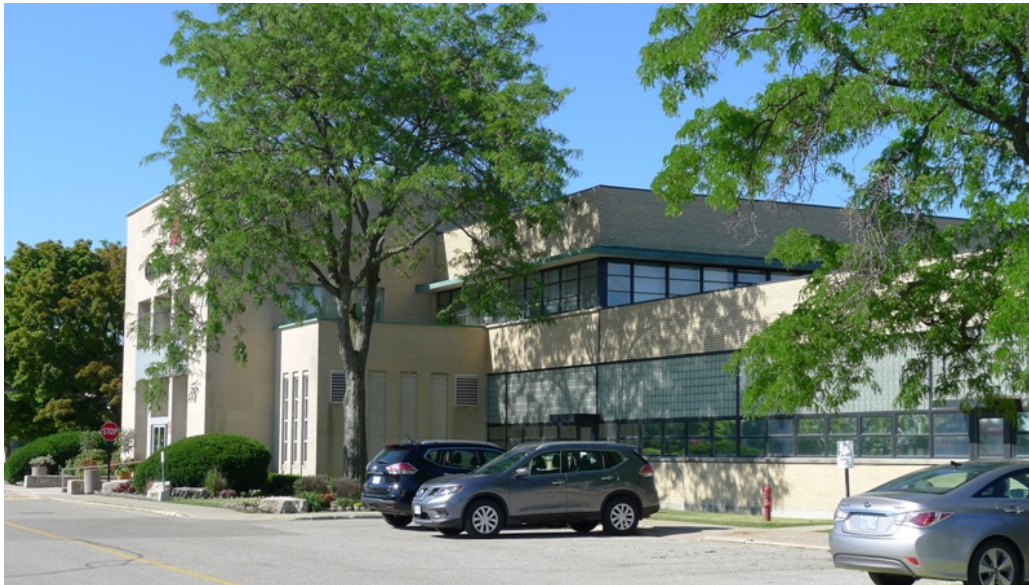
IBM Head Office and Factory, 844 Don Mills Road (1951, 1954) Clare G. MacLean architect, as photographed in 1954 ( above, Panda Associates ) and in 2016 ( below, Heritage Preservation Services ) showing the principal east elevation facing Don Mills Road
