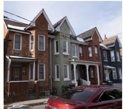
A collection of four Bay and Gable houses built c.1890 at 270-276 Sterling Road (CBCollective 2020).
