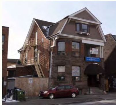
Prominent dwelling built by industrialist James Lochrie in 1894 at 1411 Bloor Street (CBCollective 2020).
