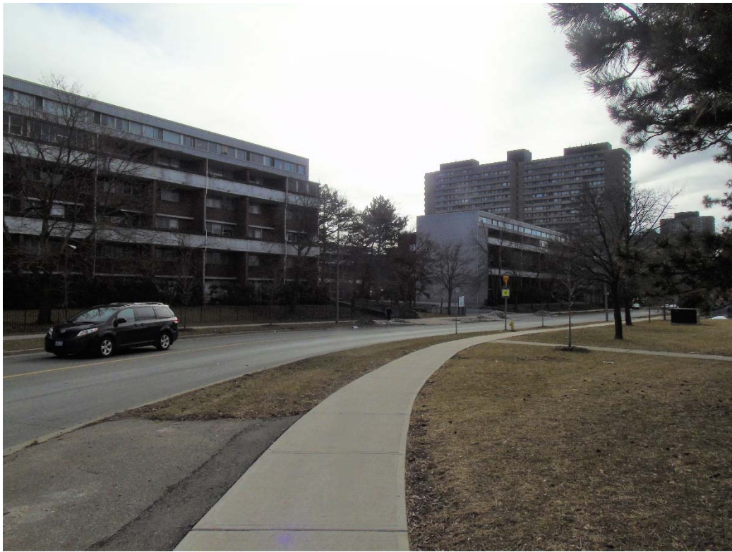
19. Housing complex at 95-155 Leeward Glenway was designed by architects Boigon and Heinonen and Raymond Mandel in 1973 as part of the Chapel Glen Development in Flemingdon Park (ASI)
