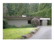
This handsome modernist residence was designed by renowned architect Ron Thom for Horace and Mary Norman. It employed simple forms of construction, with a slab on grade foundation, flat roof and flat projecting eaves. Designed on a 4 foot by 8 foot module, it is clad with sheets of plywood. The house has been maintained in original condition and the landscaping provides a beautiful and appropriate setting.
