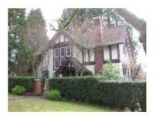
This imposing house is built in a modified version of the Tudor Revival style. It features a prominent cross-gabled roof with bellcast edges, a prominent brick chimney at the front. The detailing includes a front gabled porch, and a set of leaded glass windows that grace the main stairwell. Philip Lamson Brown (1878-1918) was a salesman, later employed by Carswell & Company Ltd.
