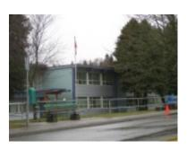
Built in response to the postwar population boom, the linear mass of this large, low-slung school building is composed of a series of interconnected structures. A one-storey block sits to the south, with a two storey block to the north. A central gymnasium is tied to both blocks by a one storey connecting wing. The present structure is the result of a building program that began in 1955, and continued with additions that began the following year.
