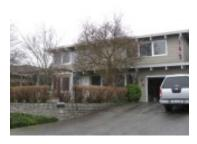
Located in Capilano Highlands, this two storey variation on a post-and-beam Lewis structure features diagonally cut beam ends and awning-swing casement windows. It was built for J. Whalley at a cost of \$16,000. A cobble stone retaining wall has been used to outline the edge of the driveway. In 1965 a recreation room was added at a cost of \$2,500. The house has been very well maintained.
