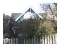
This is a well-detailed Craftsman house, with a stone foundation and a full front verandah. It occupies a prominent corner location, and features triangular eave brackets, and a front gable roof with cross gable dormers. It is unusual for being clad with drop-siding. William Turner, the first owner, ran a furniture business in Vancouver.
