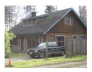
This small, compact one and one-half storey log residence is located on Dollarton Highway. The overlapped notched log corners are tapered from bottom to top. The structure has been well maintained and was recently renovated; the bottom logs have been meticulously replaced. Originally located at 2047 Dollarton Highway, adjacent to the Swedish Community Hall, the house was relocated in 1960 by T.W. Galloway and Durl Cook.
