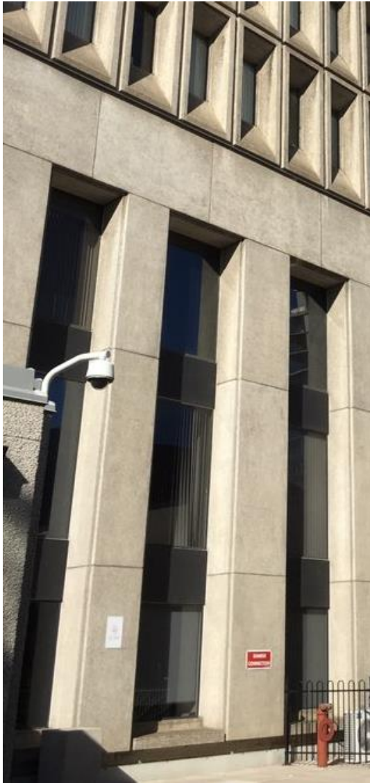
The view of exterior façade, the concrete panels look like structural columns.
