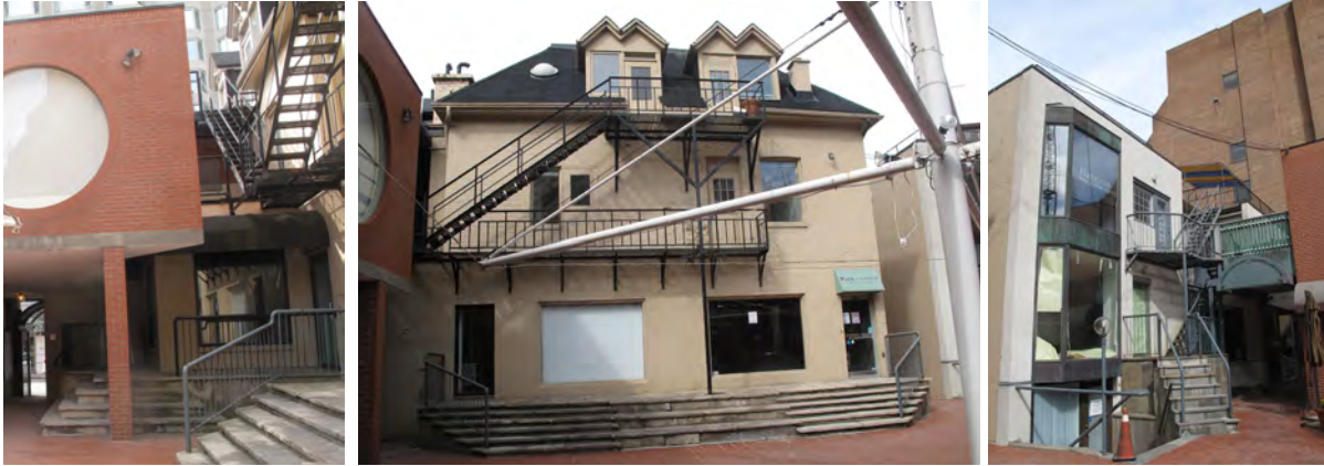
25. Views of the west courtyard walls (ERA, 2016)
