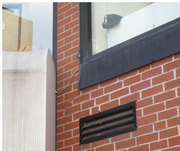
18. Detail of lifting window flashing, exposed shim and wire (ERA, 2016).
