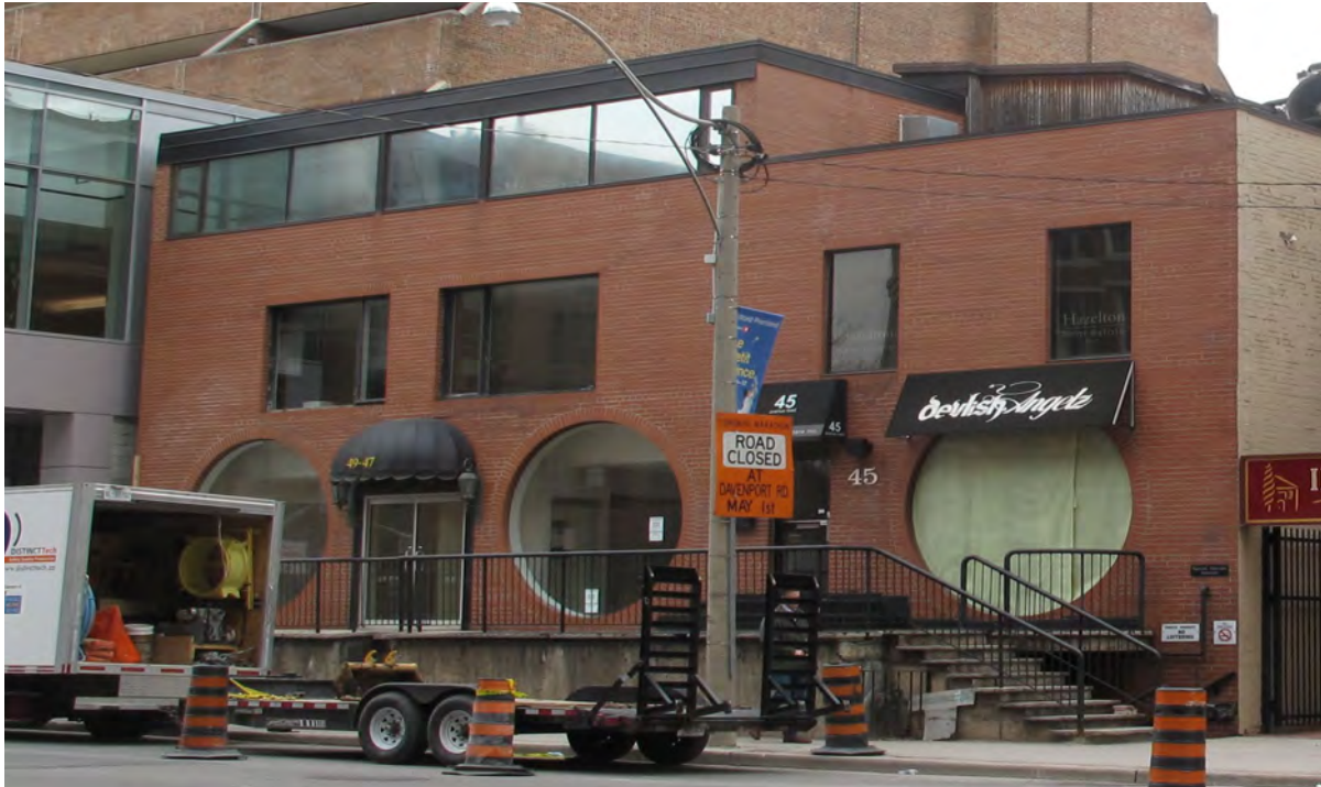
9. West Elevation of 45-49 Avenue Road - two story brick building (ERA, 2016).
