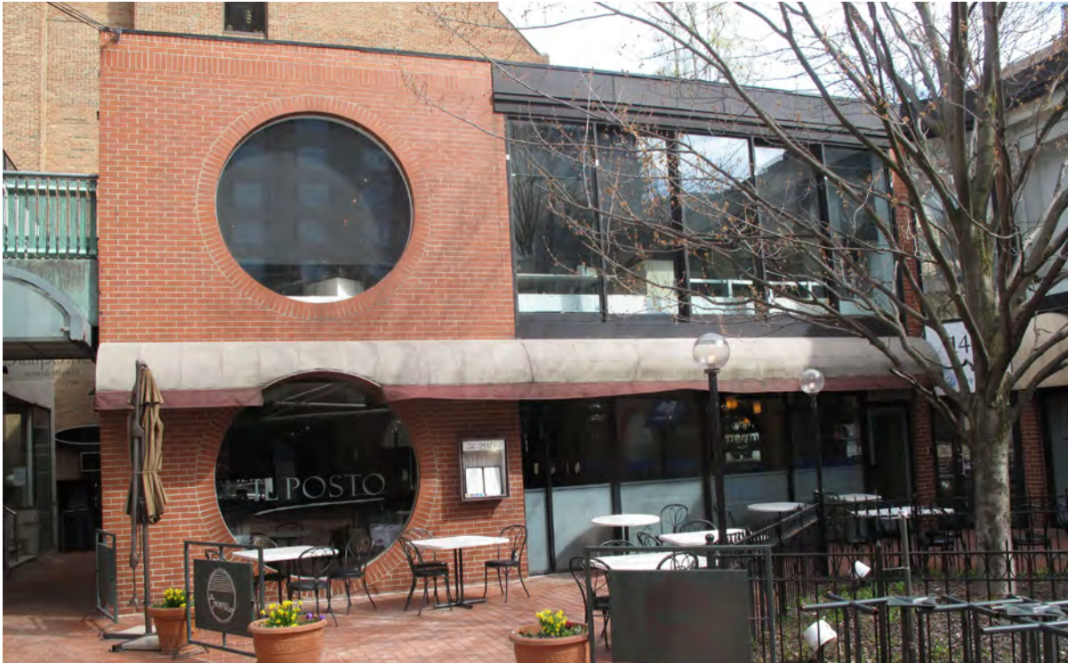
22. North courtyard wall (ERA, 2016).
