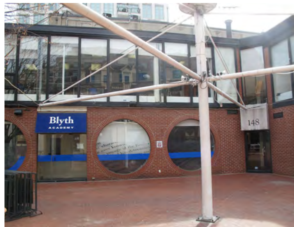
19.(b) Views of East courtyard wall (ERA, 2016).
