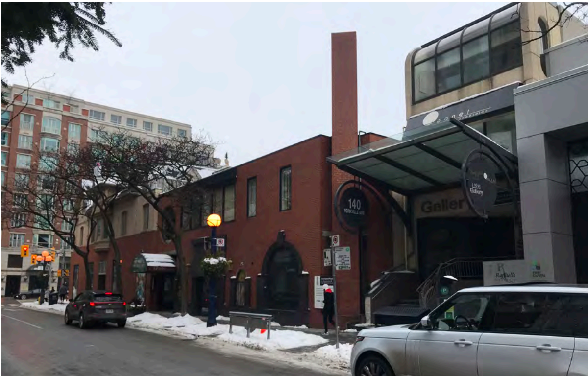
Looking west on Yorkville Avenue, showing south elevation 33 Avenue Road and 140 Yorkville Avenue (Cyprus, 2020).
