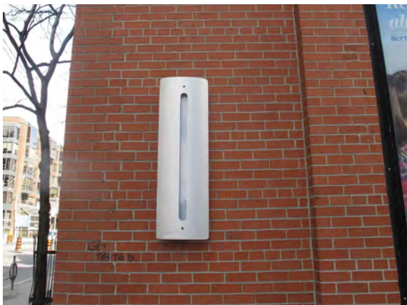
15. Detail holes and graffiti (ERA, 2016).
