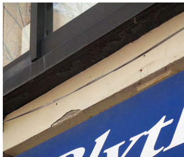
21. Detail of concrete cornice block (ERA, 2016).
