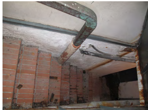
27. View of covered stairwell (ERA, 2016).
