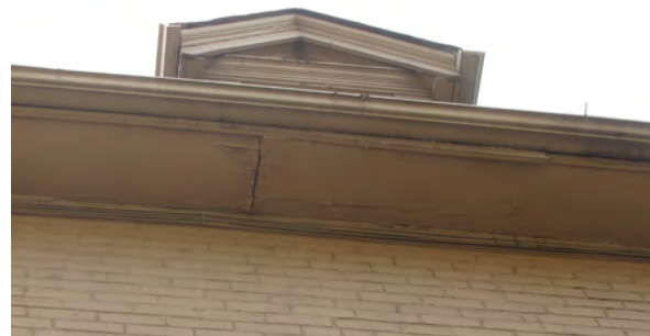
30. View soffit and one dormer (ERA, 2016).
