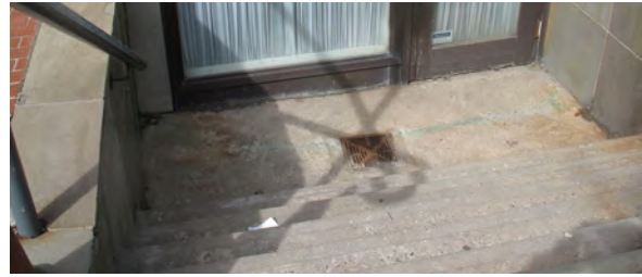
28. Detail of condition of lower level window and door (ERA, 2016).
