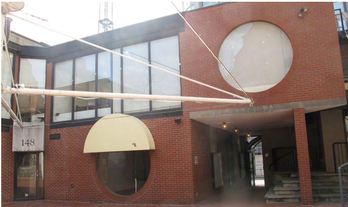
17. View of south courtyard wall (ERA, 2016).
