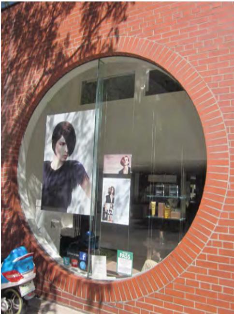
Detail of circular storefront window, Avenue Road frontage (ERA, 2018).
