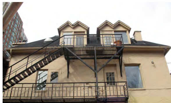
34. View of two of the dormers, roof and chimney (ERA, 2016).
