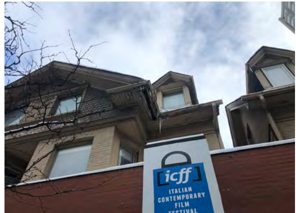
7. Detail of soffit and dormer conditions (ERA, 2020).
