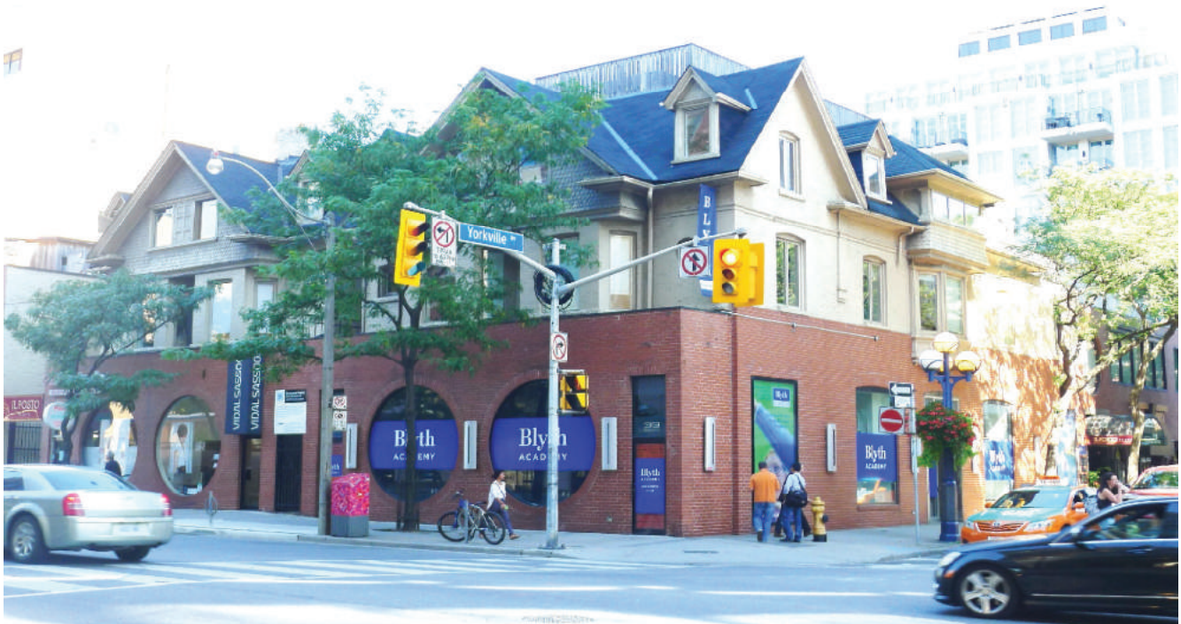
Principal (northwest) façades of York Square (Heritage Preservation Services, September 2013)
