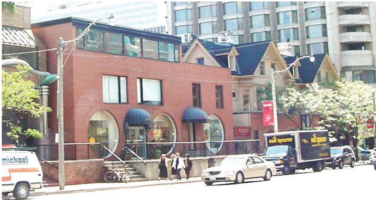
13. York Square, Three North Buildings on Avenue Road : the original buildings were completely refaced and a new third story added to two at the northern edge of the site. ( Heritage Preservation Services, October 2013 )
