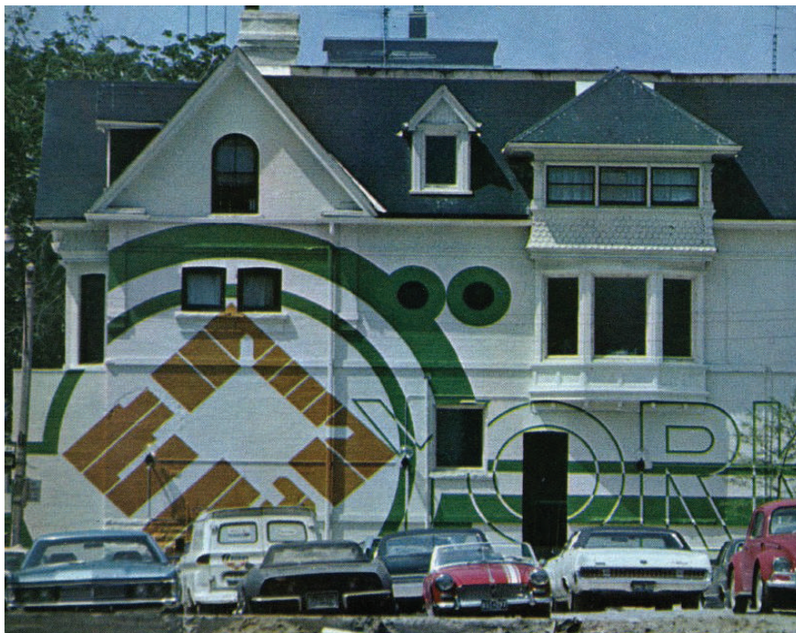
15. Supergraphics , Barrie Briscoe artist: The painting incorporates a graphic representing the plan of the complex and the letters for York Square. ( Progressive Architecture , p 148.)
