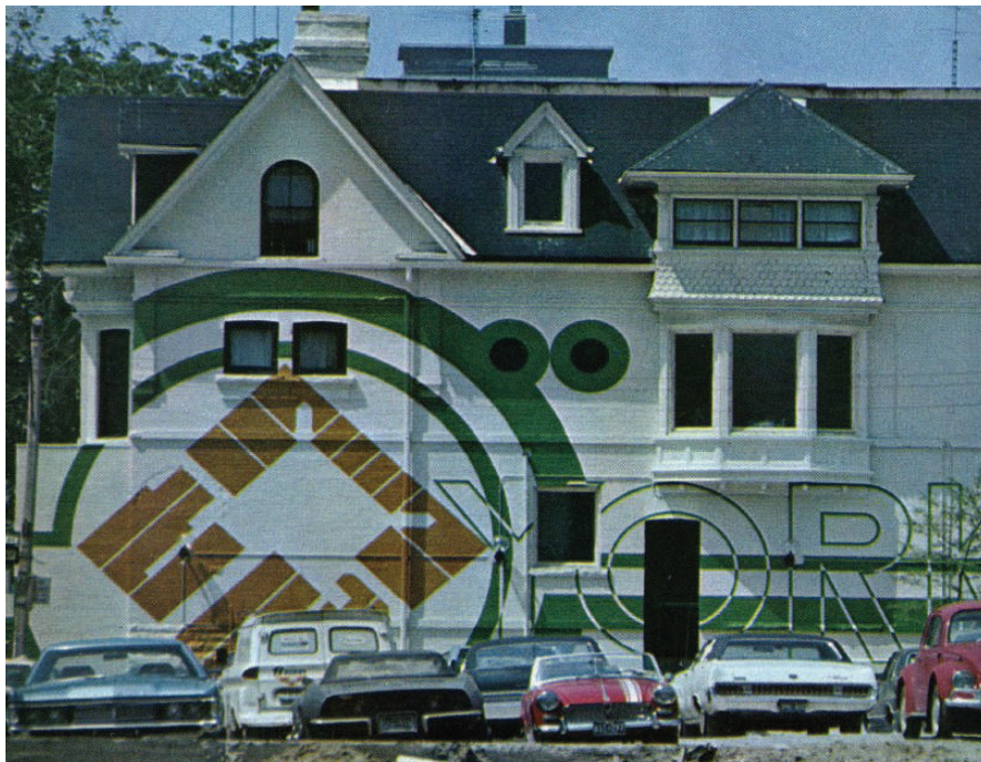
15. Supergraphics , Barrie Briscoe artist: The painting incorporates a graphic representing the plan of the complex and the letters for York Square. ( Progressive Architecture , p 148.)
