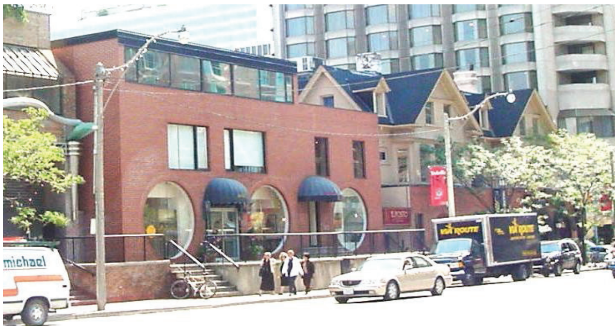
13. York Square, Three North Buildings on Avenue Road : the original buildings were completely refaced and a new third story added to two at the northern edge of the site. ( Heritage Preservation Services, October 2013 )
