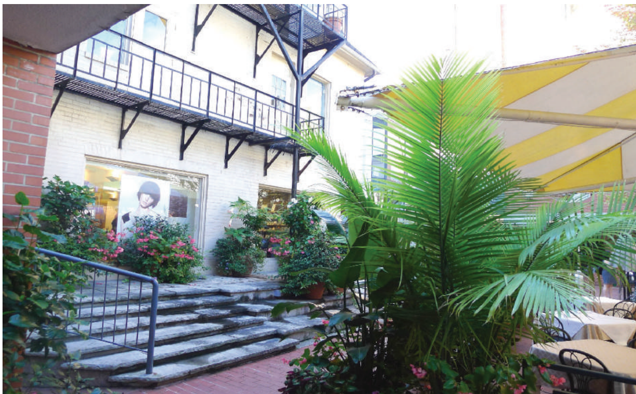
12. York Square Courtyard : Original c1900 buildings are painted and integrated into the new courtyard with new staircases and planting. ( Heritage Preservation Services, October 2013 )
