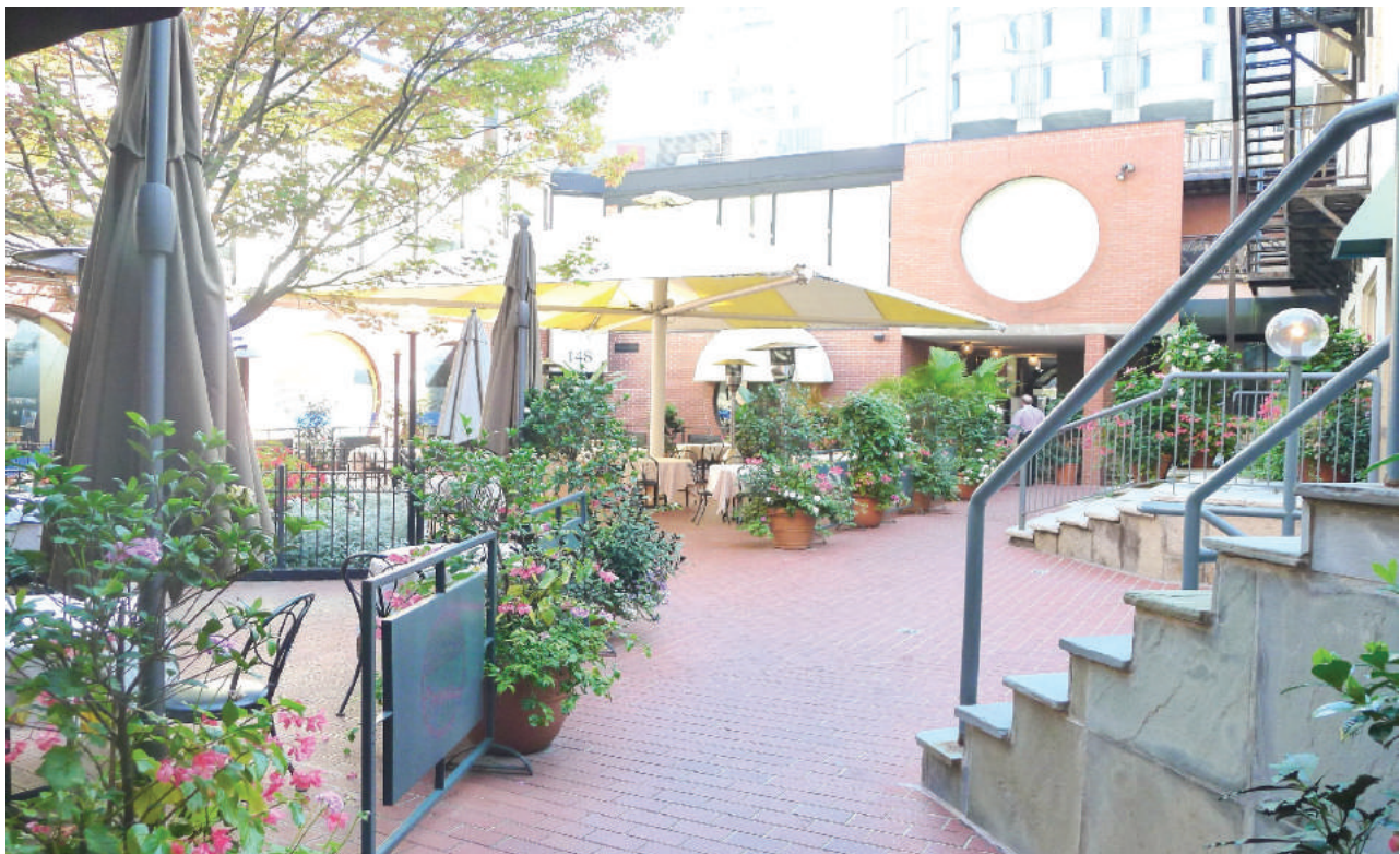
11. York Square Courtyard : showing the new building with its brick walls with circular windows and exposed concrete slabs alternating with metal framed curtain wall. ( Heritage Preservation Services , October 2013)
