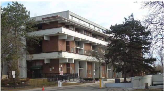
95-155 Leeward Glenway showing the north-west block, north and west elevations with expressed concrete structural beams, sheer walls and walkways and the Leeward Glenway entry driveway and access to underground parking (ASI, 2018)
