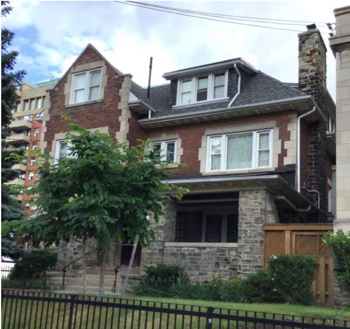
View of the principal (west) elevation of 71 Gough Avenue (Heritage Planning, 2020)
