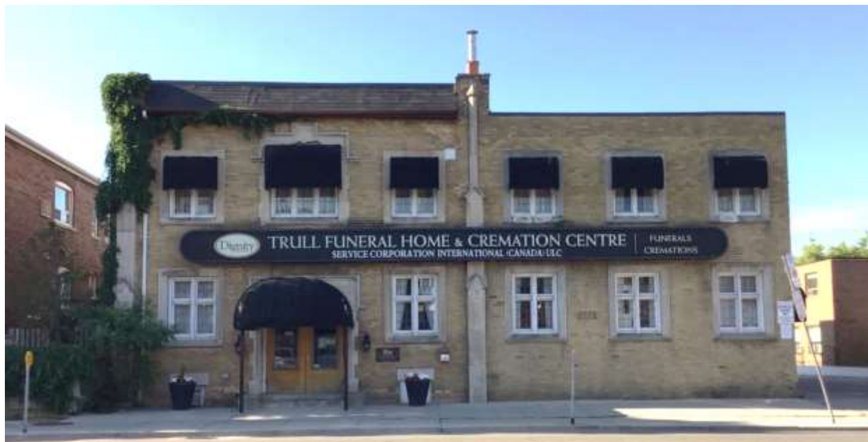
View of the principal (north) elevation of 1111 Danforth Avenue (Heritage Planning, 2020)
