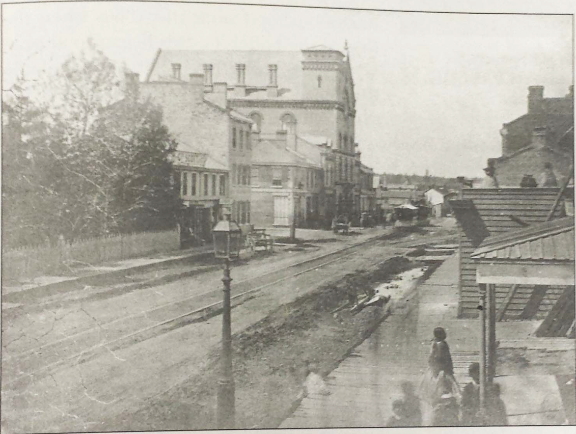
Horsedrawn trolleys had just come to Yorkville when this photo looking north on Yonge Street from near Bloor was taken. The large building served as Yorkville's town hall. It burned in 1941.
