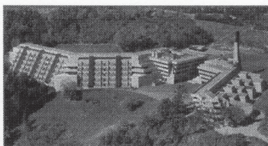
FIG. 5. JOHN ANDREWS' SCARBOROUGH COLLEGE FOR THE SCARBOROUGH CAMPUS OF THE UNIVERSITY OF TORONTO, 1965. | IMAGE COURTESY OF KEN BELL, UNIVERSITY ADVANCEMENT AND UNIVERSITY OF TORONTO PRESS.
