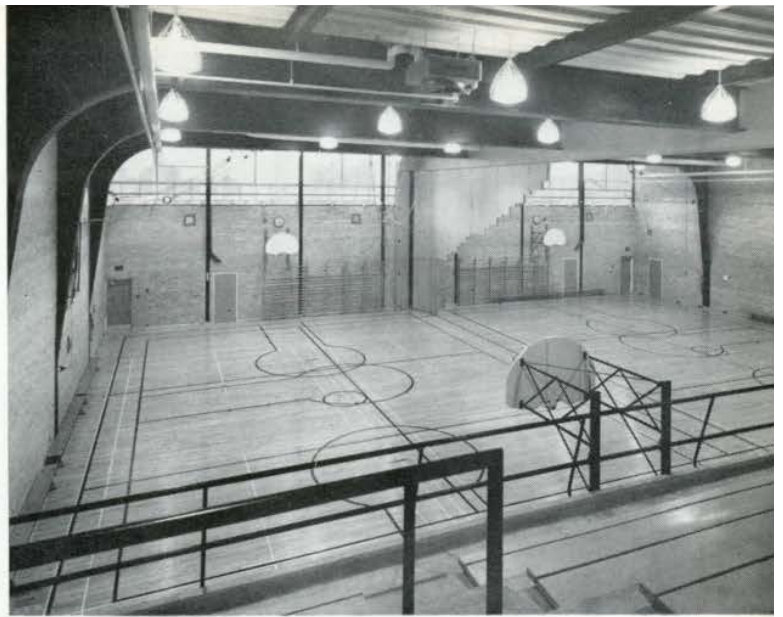
Interior of double gymnasium from gallery, showing dividing partition moving into position. Note welded steel columns and beams with precast concrete slabs roofing. Walls of natural buff brick.
