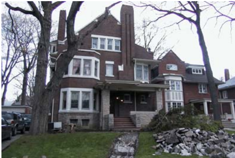
Figure 13: 112 Roxborough (1914) (C rating: good example of style, contributed to heritage character)
