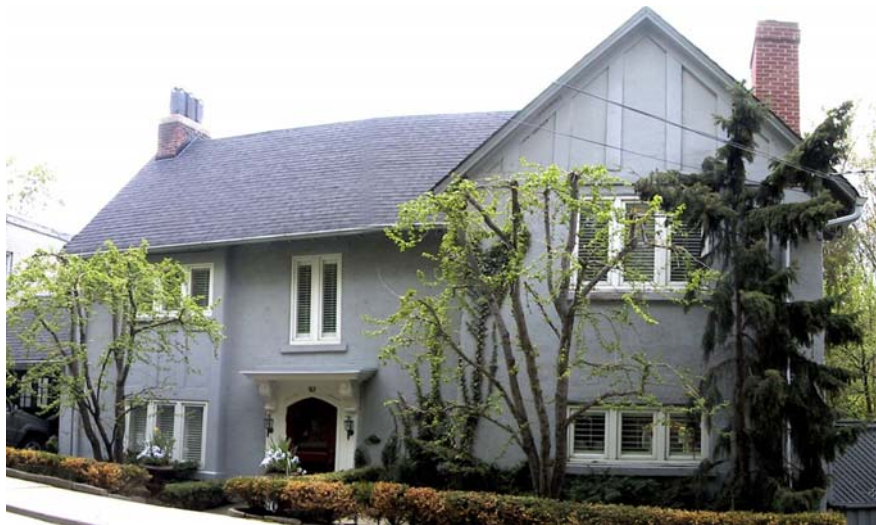
Figure 11: 83 Roxborough Drive Alfred Chapman Architect (1913) (C rating: prominent architect but appears to have undergone some alterations i.e. painting; contributes to the heritage character of the area)
