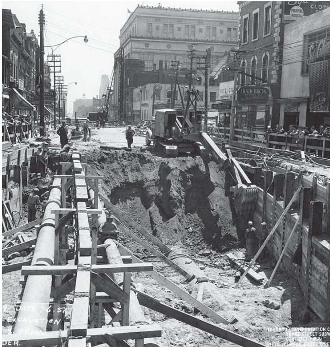
Figure 15. Photo of open-ditch subway construction from 1952, looking south along Yonge Street towards Grenville Street. Oddfellows Hall and the old Eaton's store are visible in the background.
