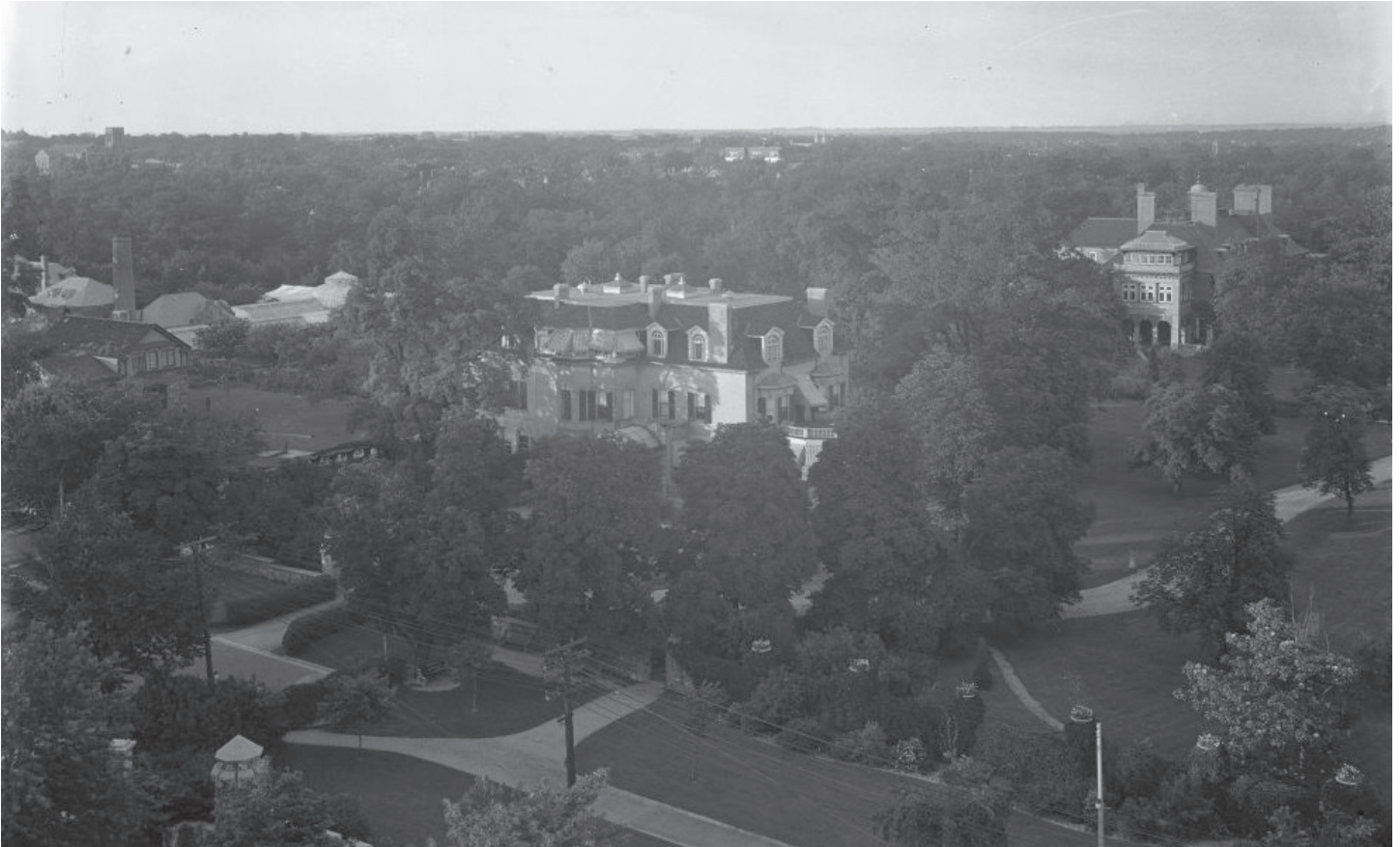
Figure 234: Looking northwest from Casa Loma tower, 1915, Toronto Archives
