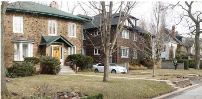
Figure 221: 369 to 371 Walmer Road
