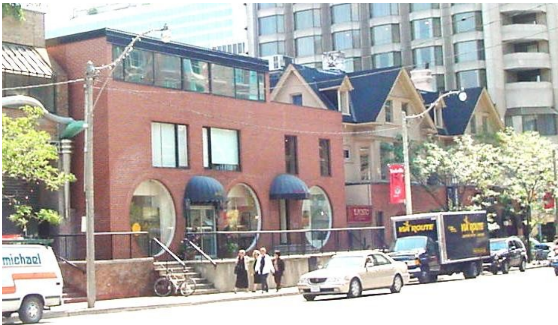
13. York Square, Three North Buildings on Avenue Road : the original buildings were completely refaced and a new third story added to two at the northern edge of the site. ( Heritage Preservation Services, October 2013 )
