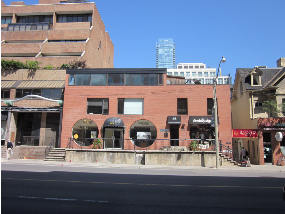
45 Avenue Road (Source: ERA Architects Inc.)
