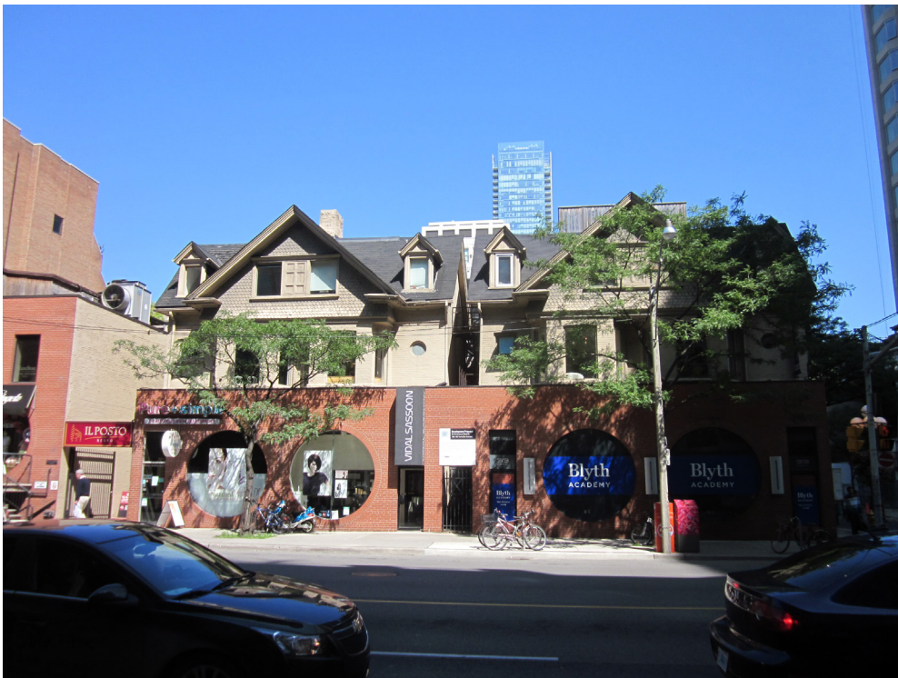
33-41 Avenue Road (Source: ERA Architects Inc.)
