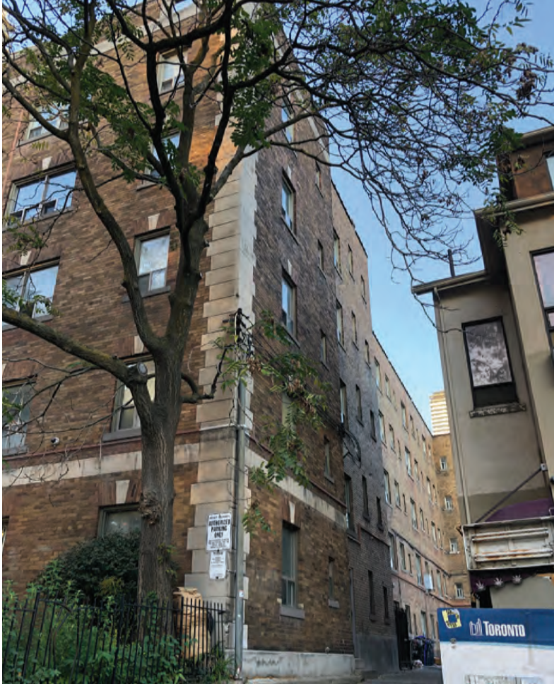
Looking towards the east elevation of 64 Wellesley Street East (ERA, 2021).
