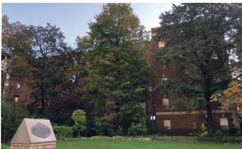
The west elevation of 64 Wellesley Street East (ERA, 2021).
