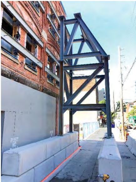
511-529 King St W – Pedestrian walkway
