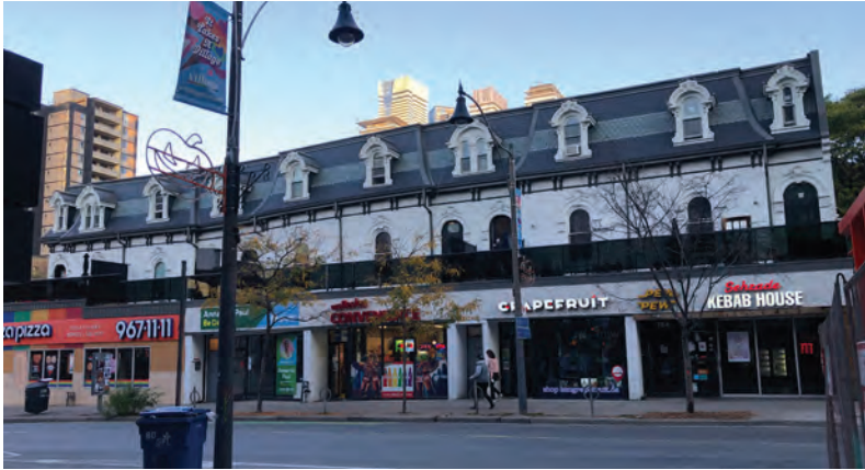
The south elevation of 68-78 Wellesley Street East (ERA, 2021).
