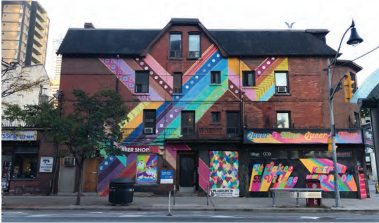
The south elevation of 552-554 Church Street (ERA, 2021).
