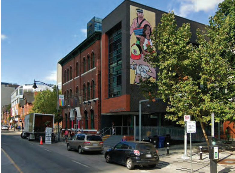
The west and south elevation of 519 Church Street (Google Maps, 2019).
