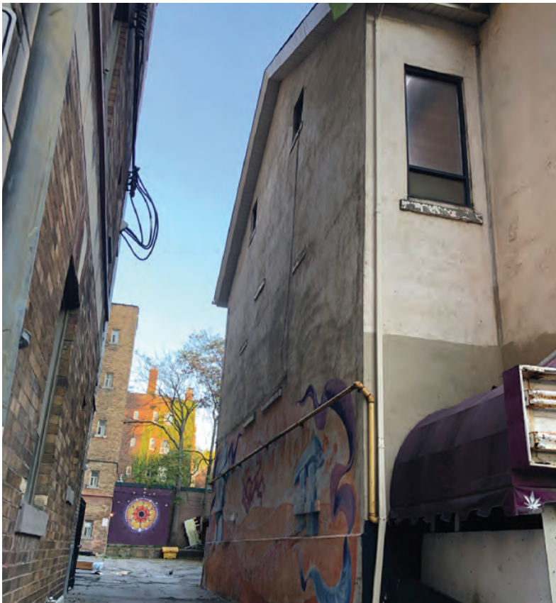
The west elevation of 66 Wellesley Street East (ERA, 2021).
