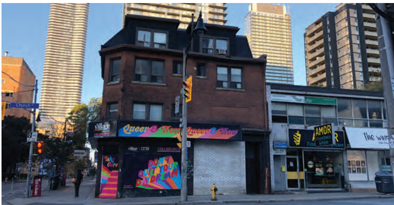
The east elevation of 552-554 Church Street (ERA, 2021).
