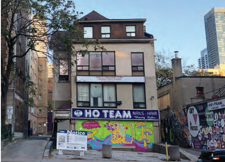
The principal (south) elevation of 66 Wellesley Street East (ERA, 2021).
