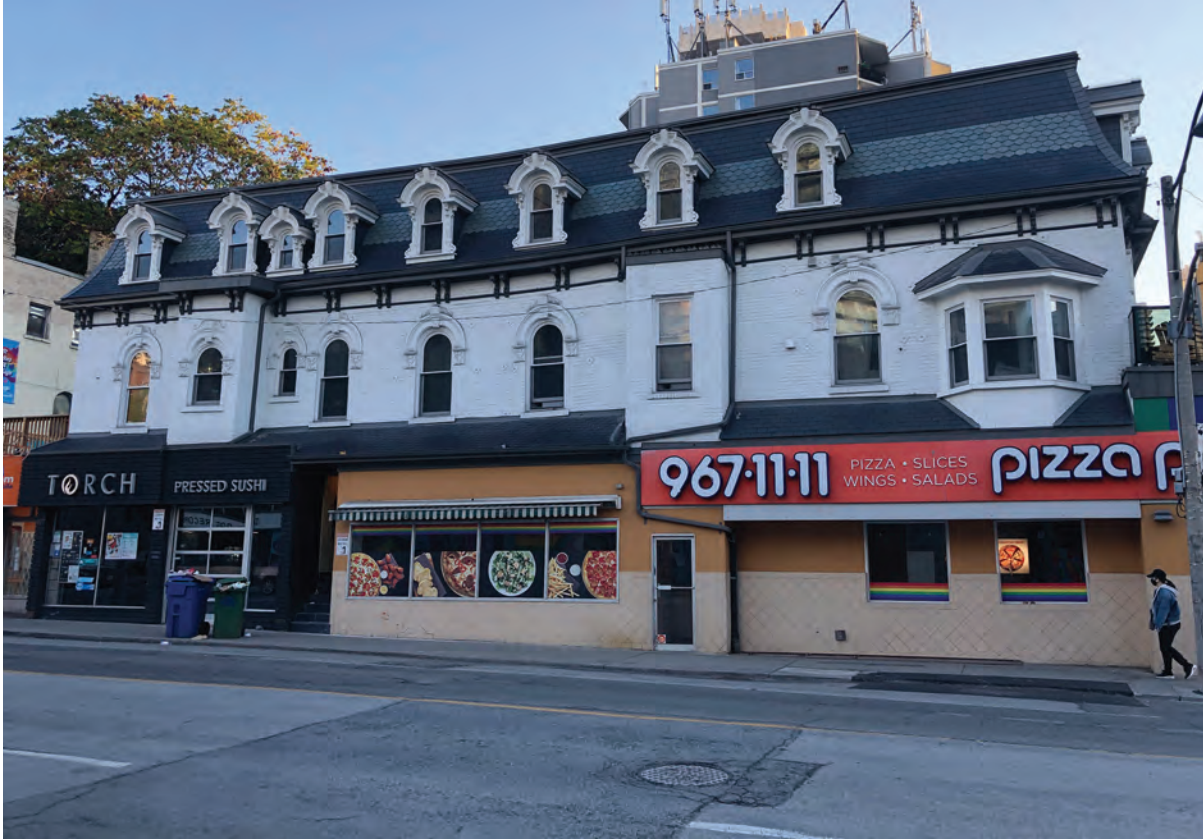
The west elevation of 68-78 Wellesley Street East (ERA, 2021).
