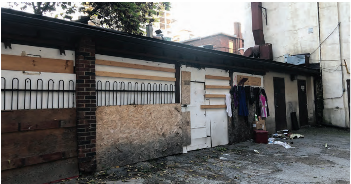
1-storey rear addition at 66 Wellesley Street East (ERA, 2021).
