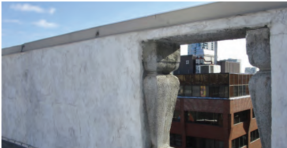
Detail of flashing on roof in good condition (ERA, 2018).
