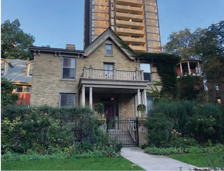
The south elevation of 56 Wellesley Street East (ERA, 2021).
