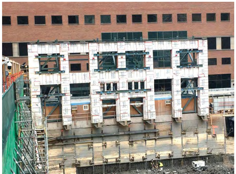
Cantilevered retention, interior needle beams
