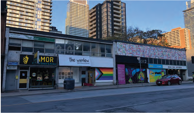
The east elevation of 560-570 Church Street (ERA, 2021).
