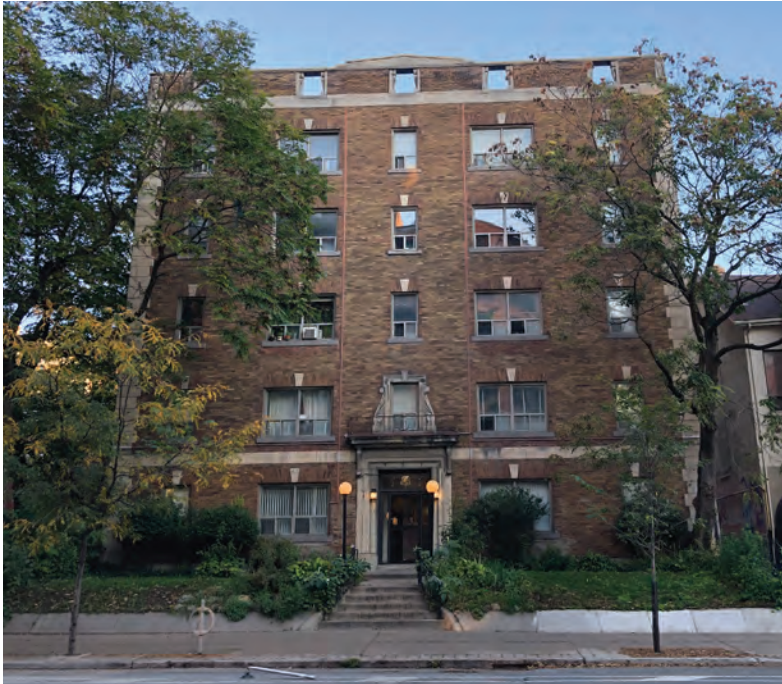
The principal (south) elevation of 64 Wellesley Street East (ERA, 2021).
