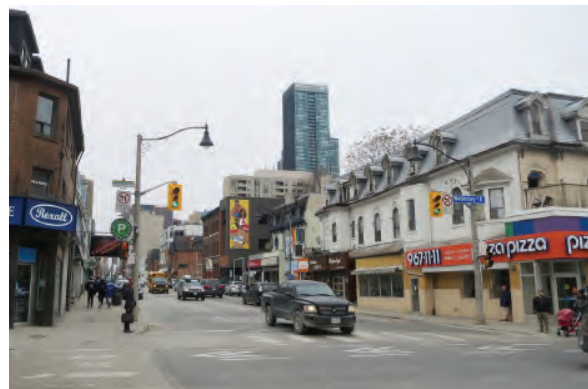
Church Street (north from Wellesley) exhibits only slightly more 19 th -century character retention (ERA 2016).
