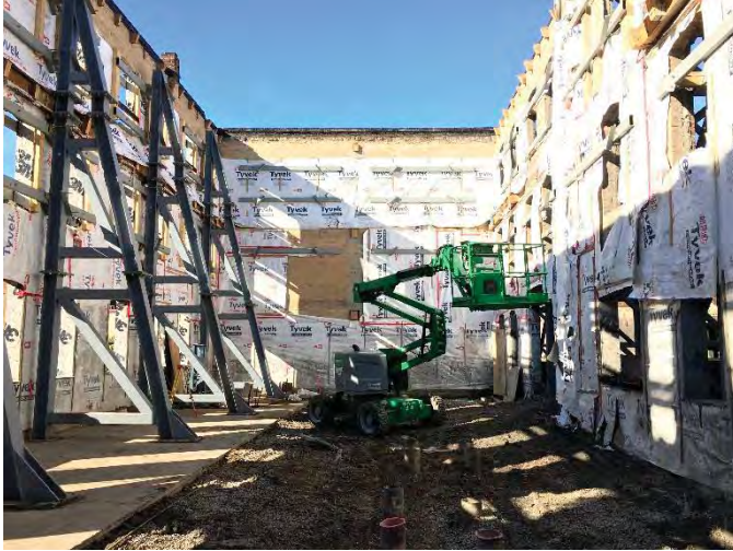
495 King St W – Interior, south elevation
