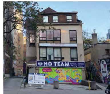
66 Wellesley Street East: 3-storey mixed use building built between 1884-1890 (ERA, 2021).
