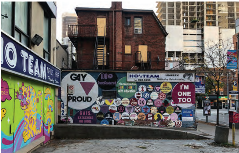
The west elevation of 552-554 Church Street (ERA, 2021).
