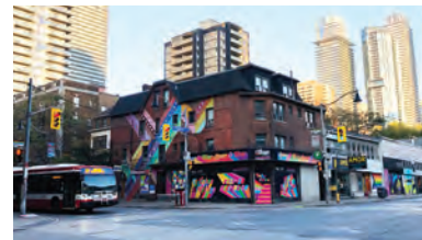
552-554 Church Street: 3-storey mixed use building built between 1884-1890 (ERA, 2021).
